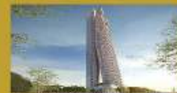
Altair, Colombo An iconic landmark of 13 lakh sq ft, designed by internationally celebrated architect Moshe Safdie.
